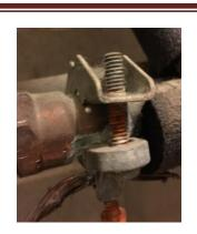
Copper pipe showing signs of corrosion
